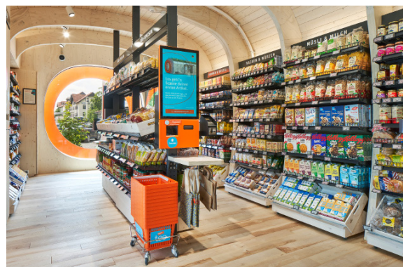
06: The interior lighting consists of two components: warm cove lighting above the product shelves and the actual product lighting with Ontero IC spotlights.
