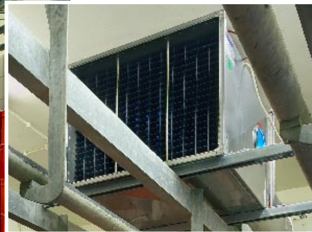
As an attachment for the cold air fan in the delivery room for fresh meat the BÄRO UV-C disinfection system reduces the bacterial count to virtually zero
