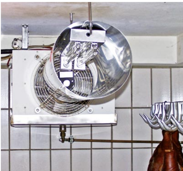
The BÄRO AirTube UV-C disinfection unit – especially for cool rooms with evaporator coolers.
